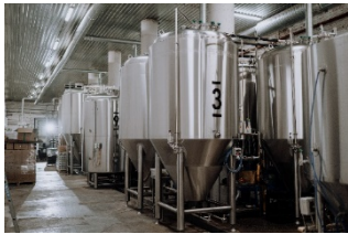
Industrial heat pump
